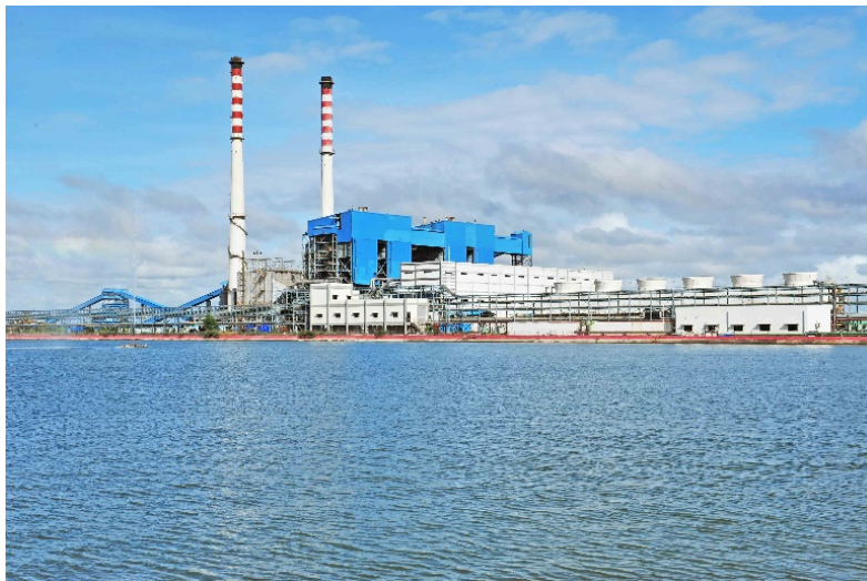
Picture of Vilayat Plant, Gujarat, India
